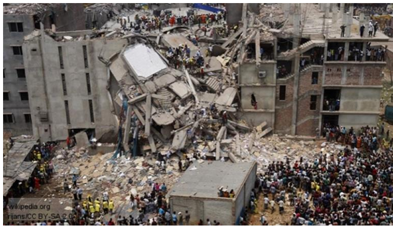
Figure 3. The process of collapse failure of the shopping center in South Korea
