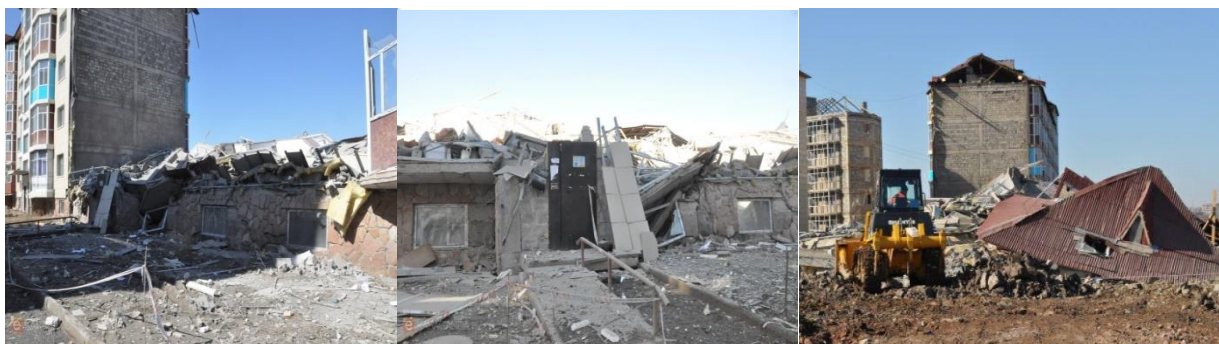
Figure 2. Collapsed houses in the Besoba microdistrict in Karaganda city
