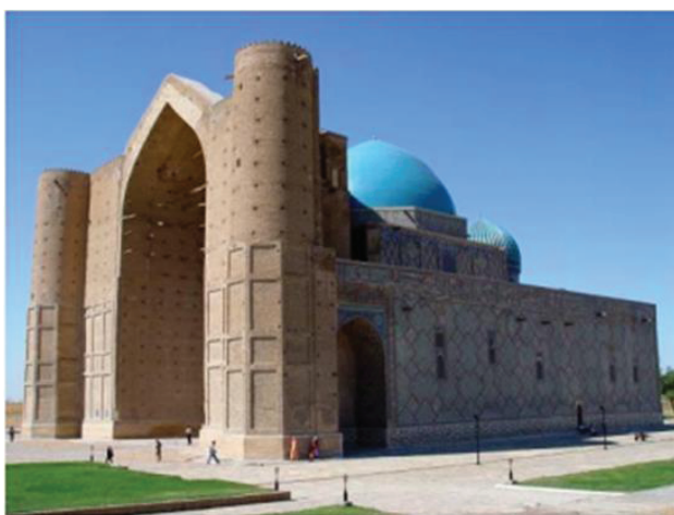
Figure 3. Schematical plan and general view of the mausoleum of Hodge Ahmed of Yassavi.
