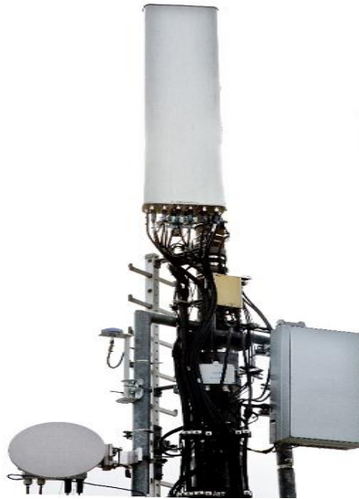
Fig. 3: The solution for the installation of a 5G technology-oriented antenna for Telefonica Deutschland
