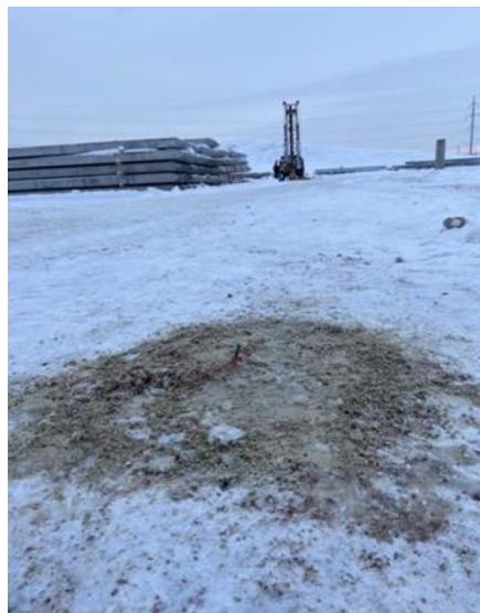
Figure 6. An antifreeze reagent on frozen ground
