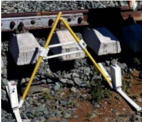
Fig.2 The second dimension along the railway under construction
