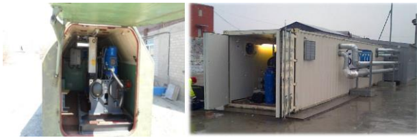
Fig. 3. General assembly of modular heat pump (MHP).
