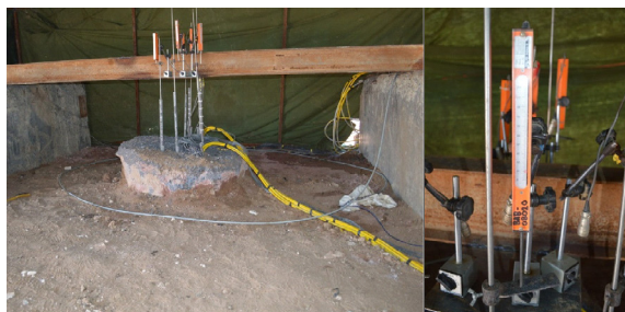
Fig. 6. Bi-Directional static load test in construction site.
