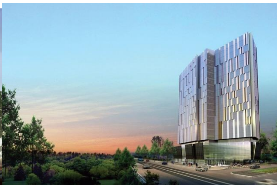
Рис. 2 Park View Office tower
